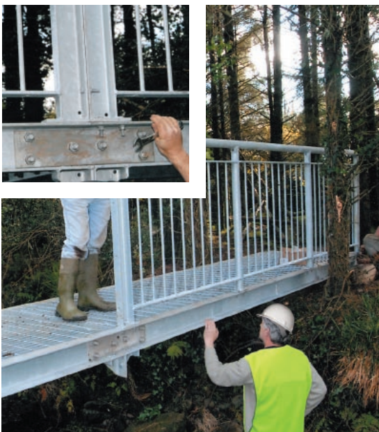
Installation (Fixing Handrail)
