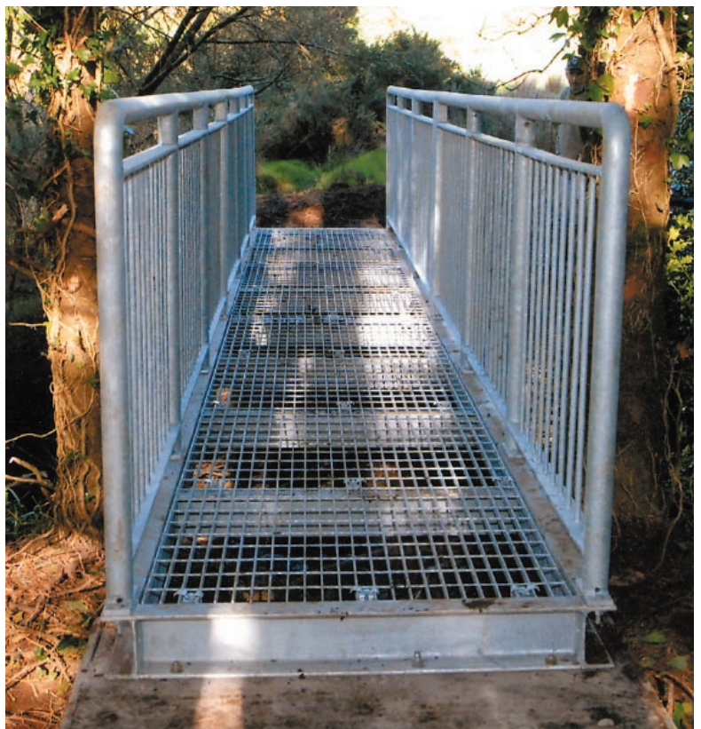
Final Bridge Structure
